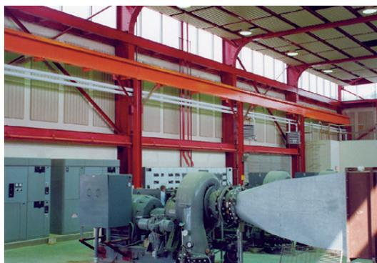
The solution involved covering about 50% of the ceiling (6,602 sq. ft.) and about 10% of the walls (2,069 sq. ft.) with the EFPs. For the ceiling treatment, three-quarters of the panels are 30 in. by 10 ft.; the remainder, 30 in. by 8 ft. On the walls, Eckel installed a mix of panels measuring 48 in. by 8 ft. and 24 in. by 6 ft. (All of these are standard EFP sizes.)
