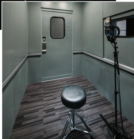
Having once been a working U.S. Mint, the original floors were built extra thick to accommodate rolling carts of precious metals and finished coins. An inherent benefit is that the existing floors help keep errant sounds from being transmitted. Normally, Eckel recording rooms are built with isolated floors that prevent the transmission of noise through vibrations.
